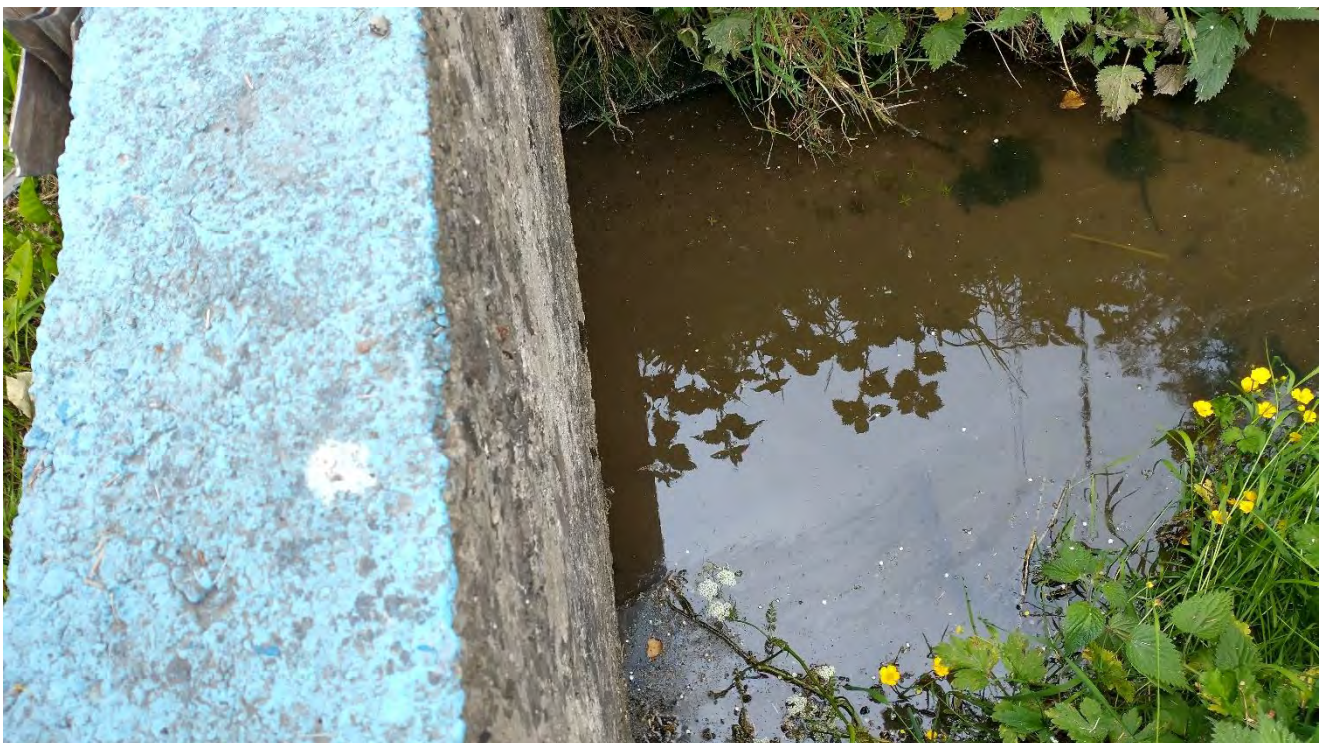
Plate 8-23: Rathnacally Stream Crossing Point/Bridge Structure
